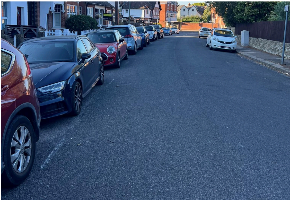
Figure D5 – Northbound on Plaistow Grove West; 07/08/26, 18:00.
