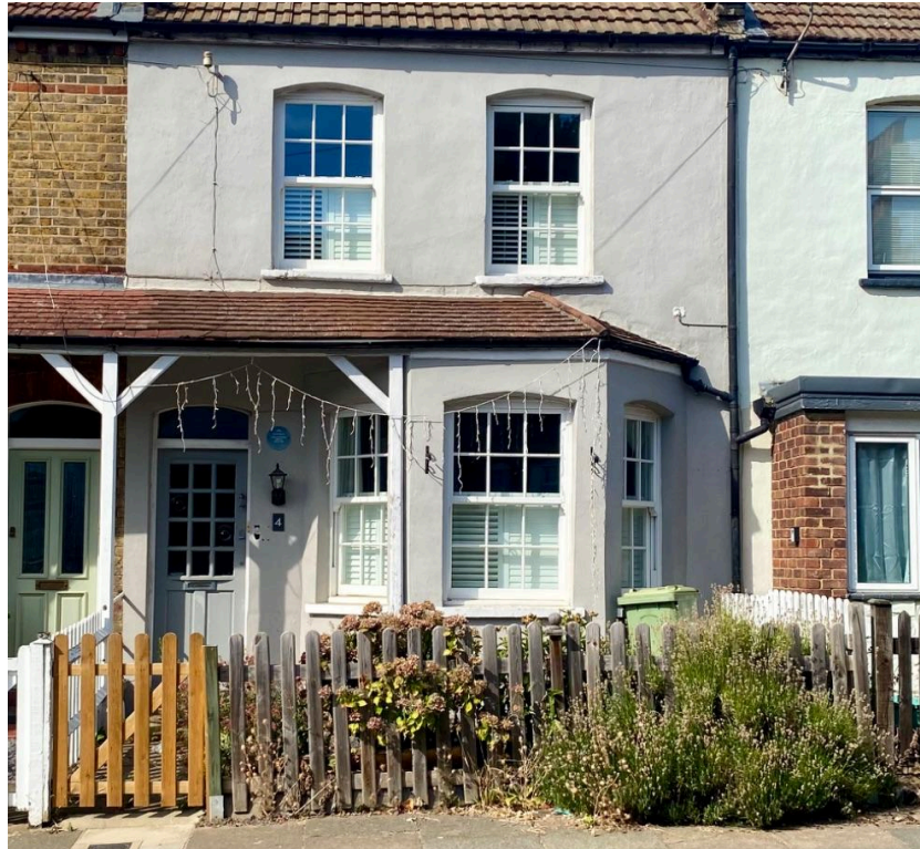
Figure 6.1 – Front view of No. 4 Plaistow Grove, showing overgrowth of planting and overall state of inattention to property (10/08/26).
